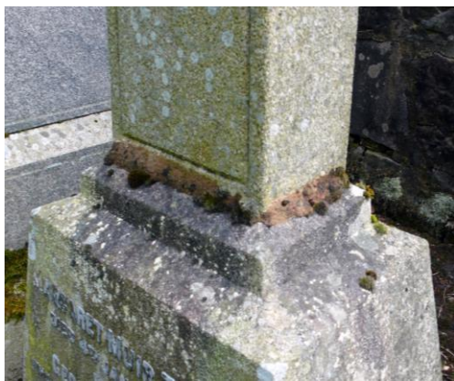
View of repair to base of Ferguson Monument
